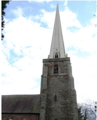
Repairs to the Spire
