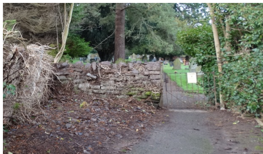
Improved entrance areas
